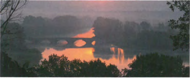
Ponte Buriano Arch Bridge / Tuscany / İtalya
