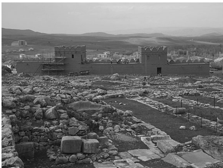
Figure 21.14 Reconstruction in progress.
