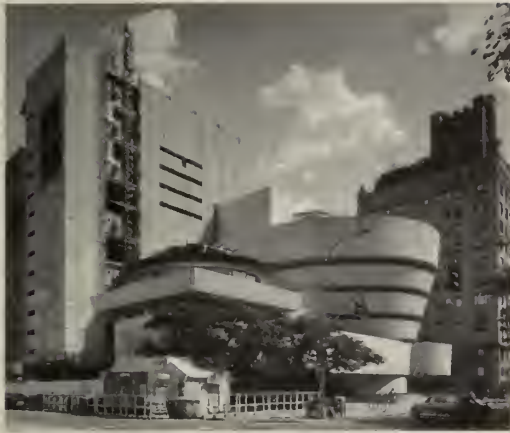
The Gwathmey Siegel addition under construction, 1990
