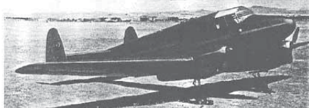
The T.H.K. 5A Light Transport (two 135 h.p. D.H. Gipsy Major engines).
