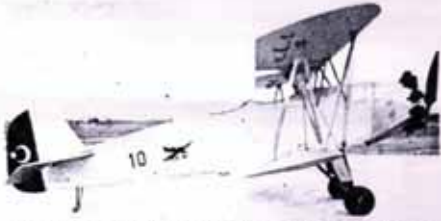
The No.D.38 Two-seat Training Biplane (100 h.p. Walter "Gemini" engine).
