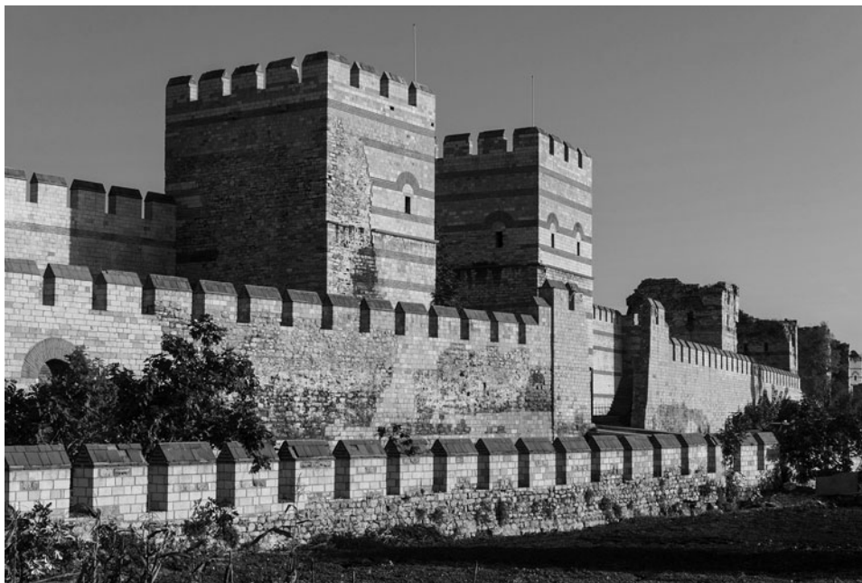
13 A reconstructed section of the Land Walls of Constantinople, which clearly shows their three-tier structure.
