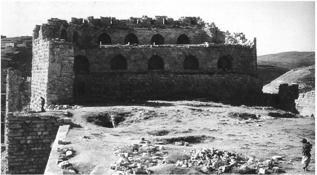
The keep at the southern end of the upper bailey of Kerak castle. This part of the complex was extensively rebuilt after Saladin captured the castle.
