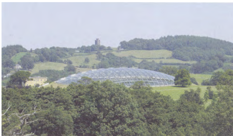
Great Glass House, National Botanic Garden, Carmarthenshire, Wales, 1995–2000.
