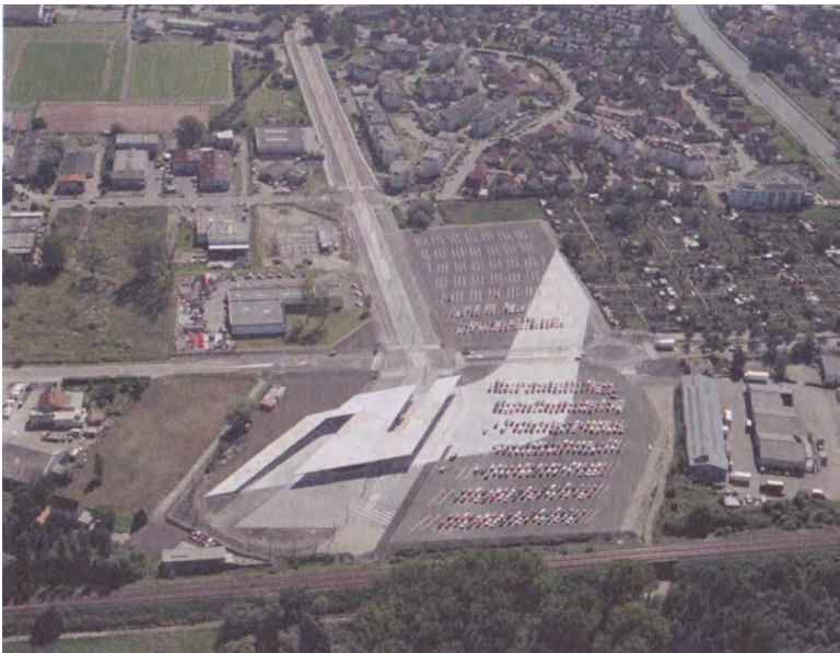
Car Park and Terminus, Strasbourg, 1998–2001.
