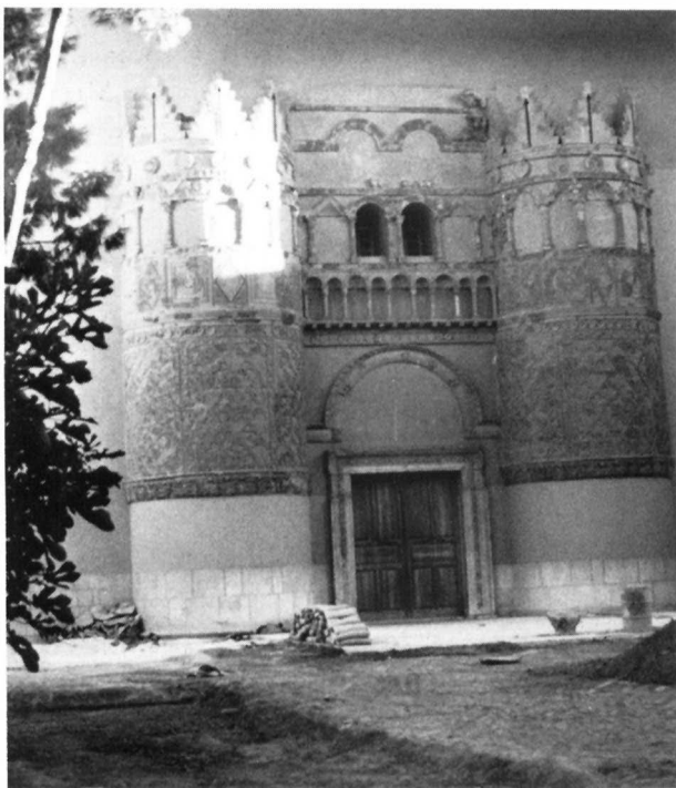
The palace or small town of Qasr al Hayr al Gharbi was built in the Syrian desert for the Caliph Hisham in 727AD. It consists of two fortified enclosures, although the defences were more decorative than functional. Here the mud-brick main gate, built on a dressed stone foundation, has been reconstructed in Damascus. (National Museum, Damascus)
