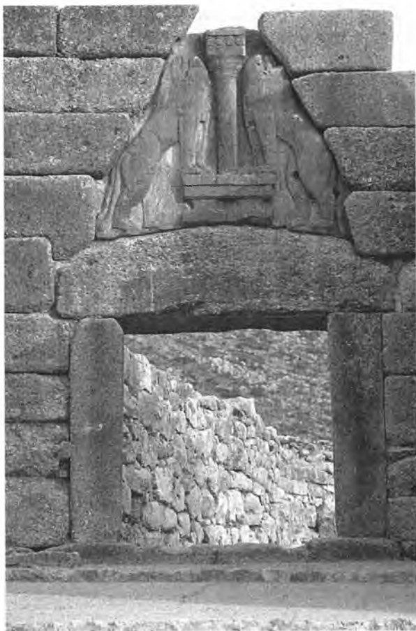
The Lion Gate of Mycenae, monumental entrance to the fortified citadel of the city. The wall around the gate is constructed of ashlar blocks. The lintel over the gate weighs 18 tons. (Erich Lessing/Art Resource, NY)
