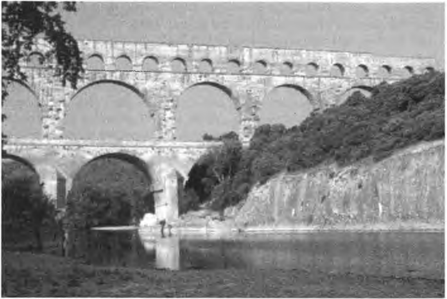
The Pont du Gard is part of a Roman aqueduct constructed in the first century A.D. to bring water to the city of Nîmes in France. (Vanni/Art Resource, NY)
