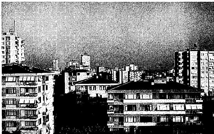
9.7. Proliferation of concrete slab block apartments in Istanbul. (Photograph by the author.)
