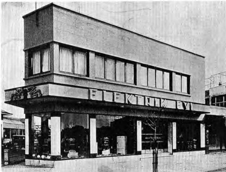
Fig. 3.13. Offices of the Société Anonyme Turquie d'Installation Électrique (SATIE) in Fındıklı, Istanbul (1934), by Sedad Hakkı Eldem, displaying the Corbusean principles of flat roof, horizontal band windows, pilotis , and free plan. Figure 3.14. "House of Electricity," a store for electrical appliances in Kadıköy, Istanbul (1937), by Rebii Gorbun. The plain "cubic" volume of the building, the transparency of the ground floor, and the use of reinforced concrete mushroom columns on the lower level are some of the most conspicuously "modern" features of the building.
