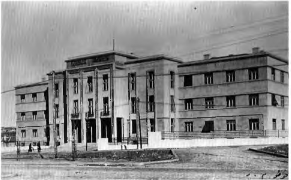
Fig. 1.15. Coexistence of the “national style” and the “New Architecture” in Ankara at the end of the 1920s: two government buildings completed at the same time along prestigious Atatürk Boulevard. Top: Ministry of Foreign Affairs (1927), by Arif Hikmet Koyunoğlu. Bottom: Ministry of Health (1927), by Theodor Post. Postcards, circa 1930.
