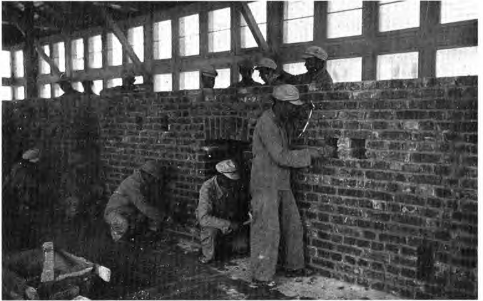
Fig. 4.14. Training workers in masonry ( top ) and brick-laying ( bottom ) at the newly established Building Trade School in Ankara, which started its program in 1932. Photographs circa 1938.
