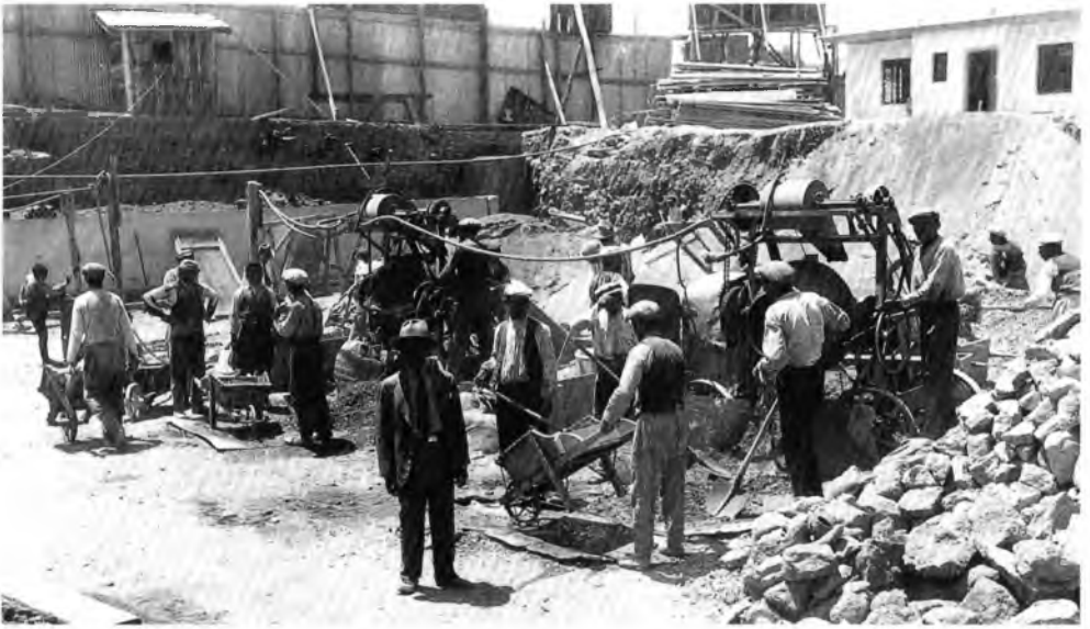
Fig. 4.13. Construction of the Sümerbank building, Ankara (1937). The photograph reflects the primitive conditions of the construction industry even for a building of this size and importance.
