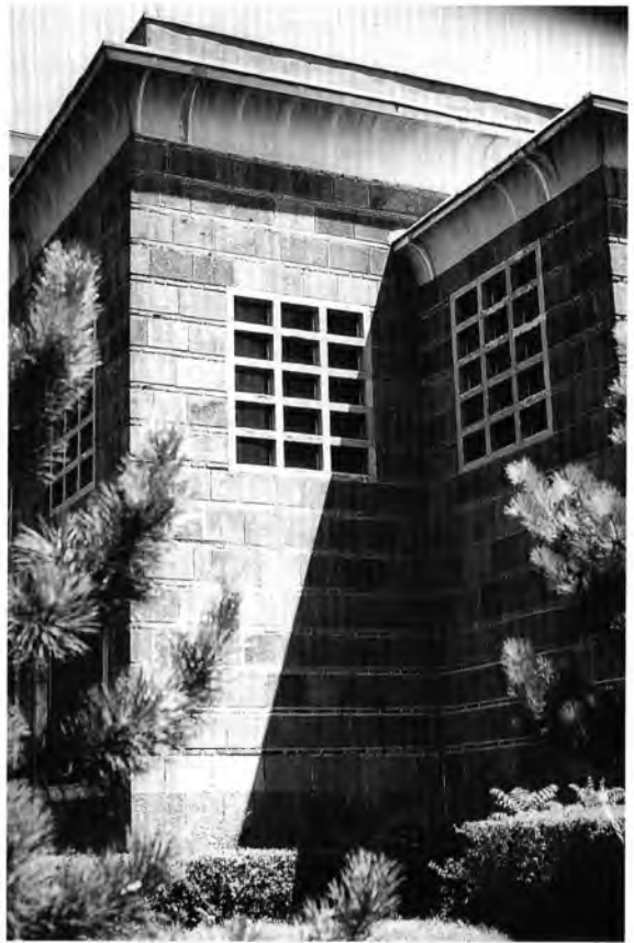
Fig. 6.11. Detail of the Faculty of Humanities, Ankara (1937), by Bruno Taut (see also fig. 2.9). The alternating courses of stone and brick are used in the manner of traditional Ottoman walling techniques.
