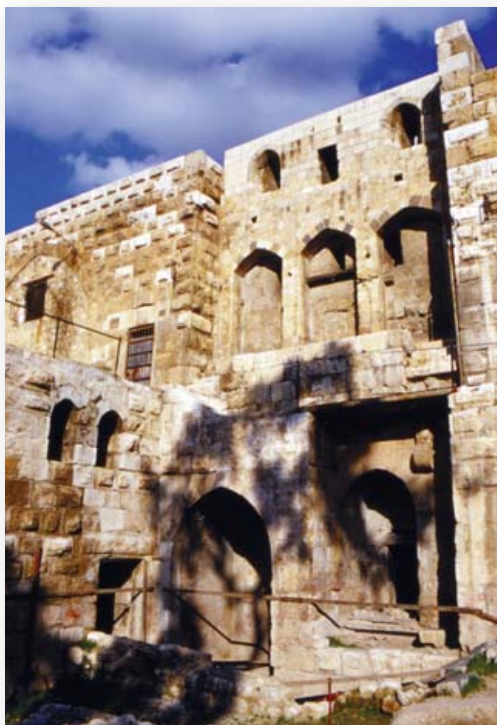
Interior of the eastern wall of the Citadel of Damascus, largely dating from the early 13th century. It includes large chambers that were used as barracks, workshops and storage rooms throughout the Mamluk period. (Author's photograph)
