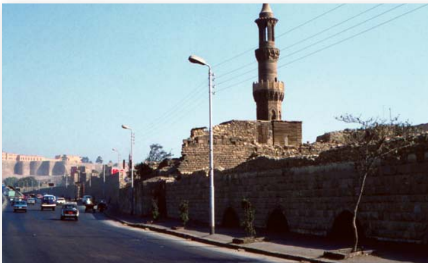
The remarkable aqueduct that brought water from the Nile to the Citadel of Cairo was built in steps, each originally marked by a saqiya water-mill. It was re-activated in the first half of the 14th century to bring water to a Mamluk palace complex at the southern end of the citadel. (Author's photograph)
