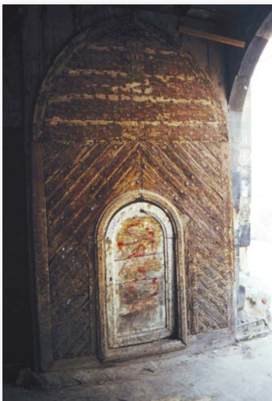
Massive wooden door leading into the courtyard of the Bayt al-Ijani, incorporating a smaller door for pedestrians. (Author's photograph)
