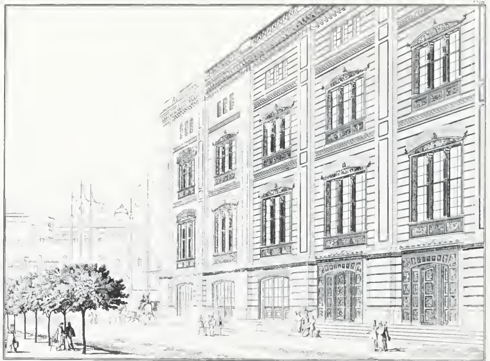
3.7 Karl Friedrich Schinkel, Bauakademie, Berlin, 1836. Note that the centers of the rafters cor- respond to the centers of the indented cor- bels on the cornice of the building.
