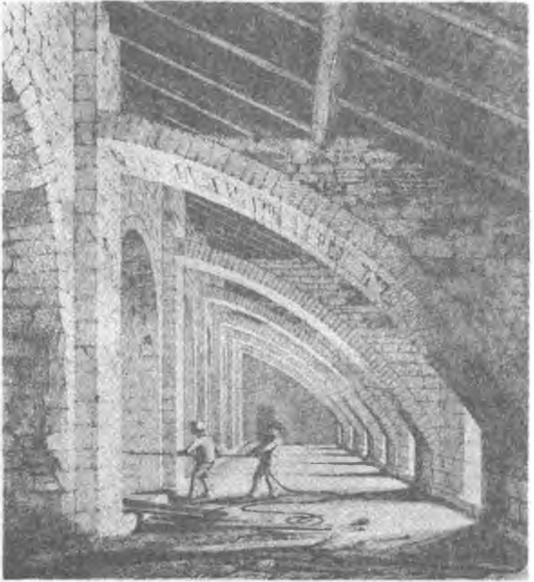
Resim 28: Durham Katedrali, gizlenmiş uçan payandalar, on birinci yüzyıl sonu. (R. W. Billings, Architectural Illustrations and Descriptions of the Cathedral Church of Durham , London, 1843).
