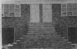
ground-level, Two-Block House, Jersey City, N. J.
