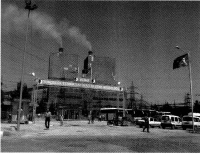
Tunçbilek Termik Santrali
