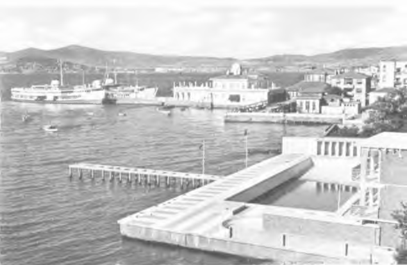
18. İskele binası, vapurlar ve yeni yapılanma (1970'ler). The terminal building, ferries berthed at the pier, and a new construction site in the 1970s.
