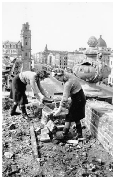
Figure 65. Two young women repair the roof of Gostiny Dvor on Nevsky Prospect in the summer of 1944. TsGAKFFD, Ar99069 (Miscellaneous collection).
