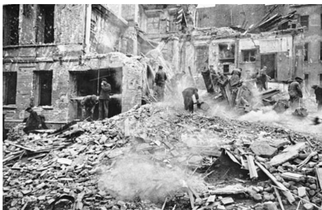
Figure 29. Bomb damage, September 1941. TsGAKFFD, Ar17086 (Box 305).
