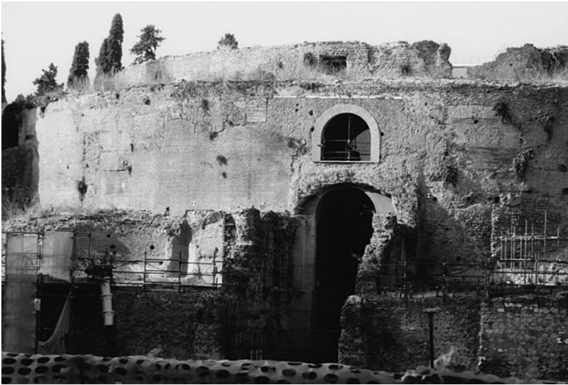
Figure AI.7 Augustus' Mausoleum undergoing repair and restoration in 2012. This photo shows the single entrance and the exposed brick and stone work of the circular drum. The superstructure has disappeared and no-one can say how the upper sections of the Mausoleum were originally constructed. Like Hadrian's Mausoleum on the opposite bank of the Tiber, it was once converted into a fortress but went out of use in the medieval period, when gardens were laid out inside the top of the drum. In the later twentieth century this monument was seriously neglected and had become somewhat overgrown and desolate, so the restoration is very heartening.
