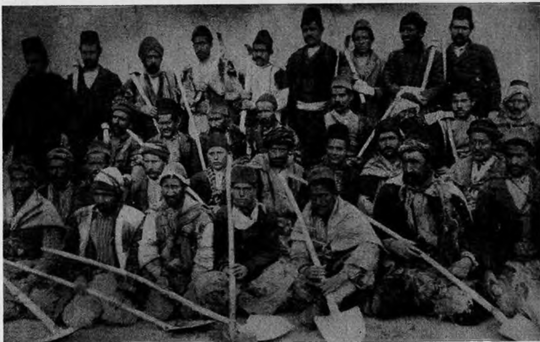
Armenian Trench Diggers
